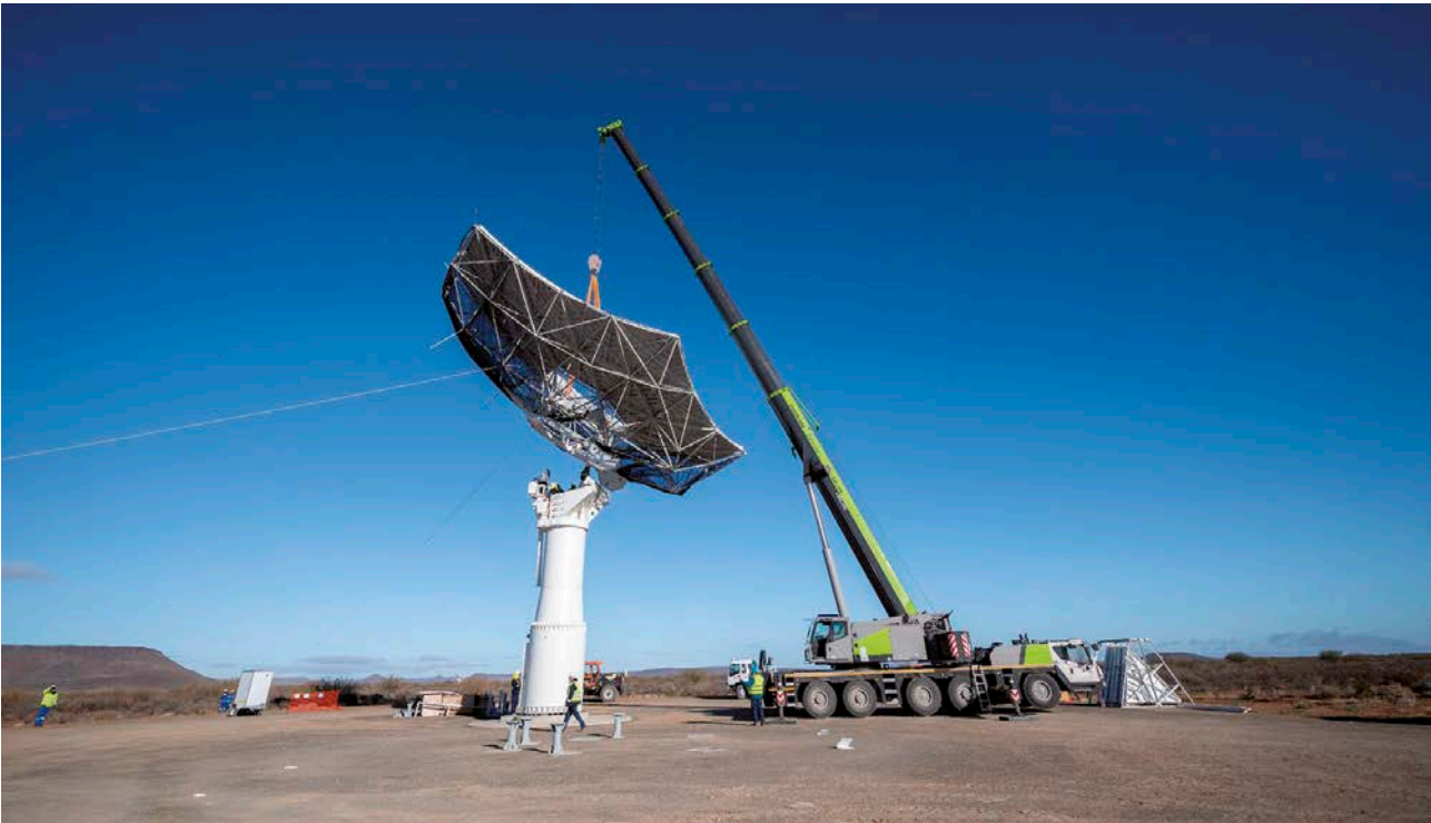
SKA-MPI, the Max Planck Society funded prototype dish, being assembled at the SKA-Mid site in South Africa. Credit: Nasief Manie/SARAO
